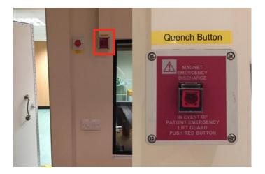
The magnet field will take approx. 30-40 seconds to collapse. Do not take anything ferromagnetic into the magnet room until it has been confirmed the magnetic field has dissipated (the object will no longer be attracted to the magnet).
